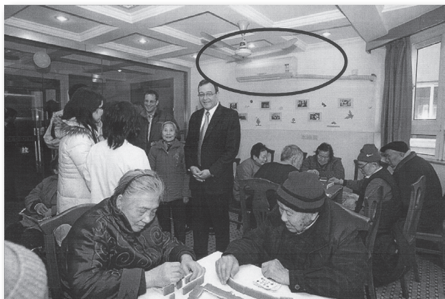
A heating system was installed on every floor of the pensioners' club. Uri Gutman, the Consul General of Israel in Shanghai, stands in the center
