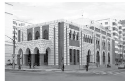
New Synagogue - restoration almost complete
